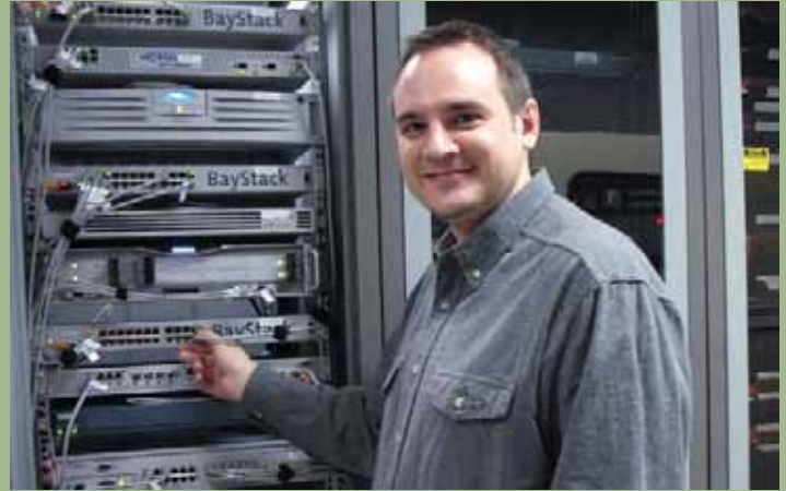
A member of the Alberta Blue Cross Networks, Communications and Security Services team, Richard Hanak is helping to develop network systems that make sense for Alberta Blue Cross customers and Alberta's health service providers.
